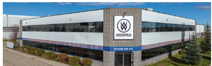
REV Engineering Ltd leased 88,000 square foot at 5616 80th Avenue SE.
